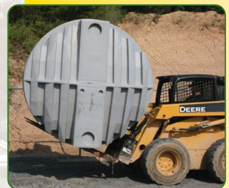
Light-weight modules can be handled with small excavator or skid steer loader.
