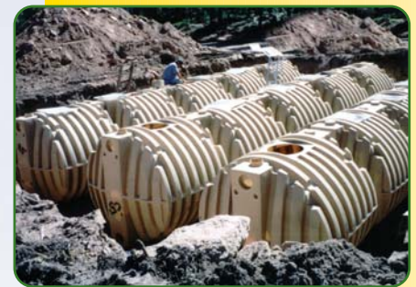
Modular tank design allows for storage capacity from 2,000 to 30,000 gallons.
